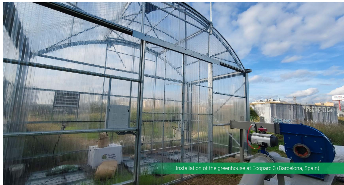
Installation of the concentrator and percolating biofilter at Ecoparc 3 (Barcelona, Spain).
