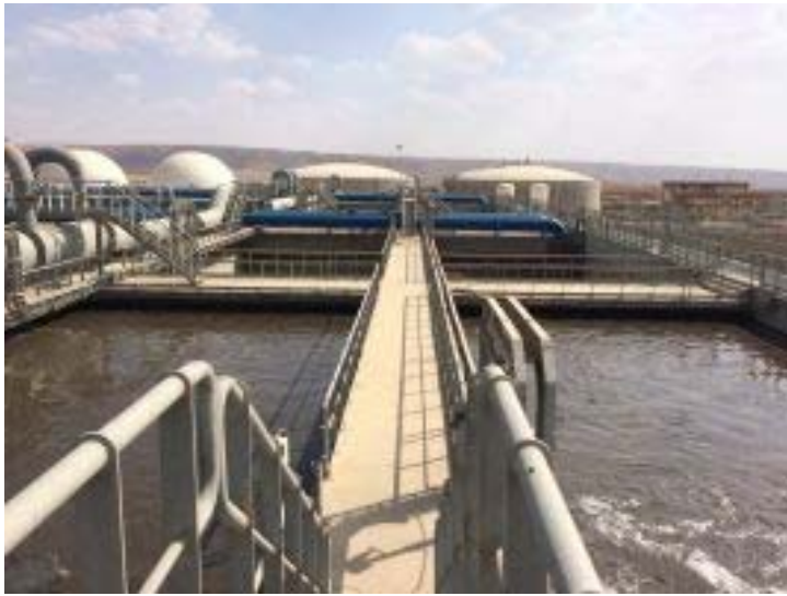
FCC Aqualia signed a contract to build the Abu Rawash wastewater treatment plant in Egypt
