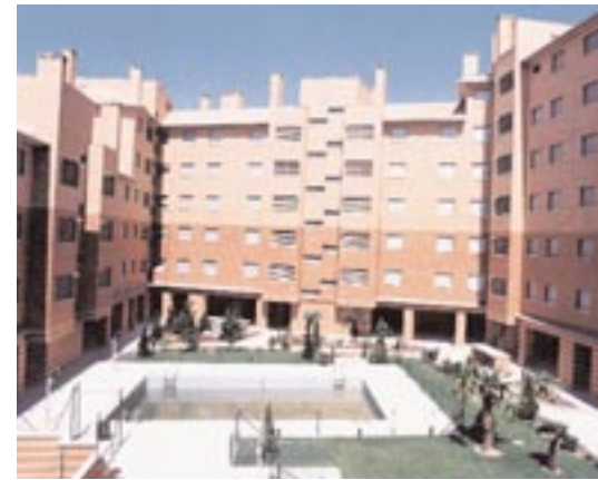
Santa Rita II, block of flats. Madrid
