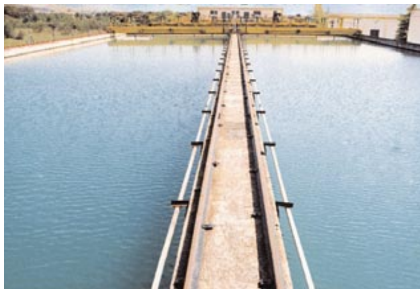
Drinking-water treatment station in Talavera de la Reina. Toledo
