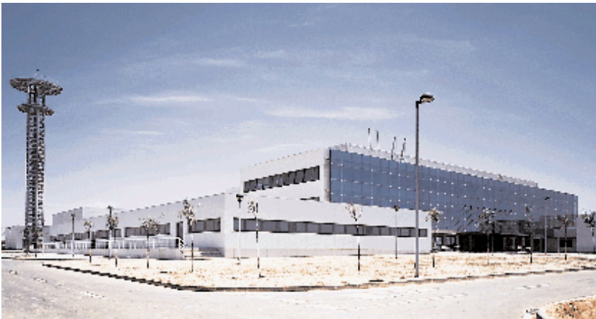
Barcelona Airport. Control centre in Gavá
