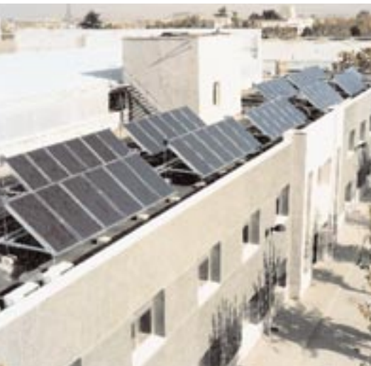
Exterior of the Villaverde Vehicle Yard. Madrid
