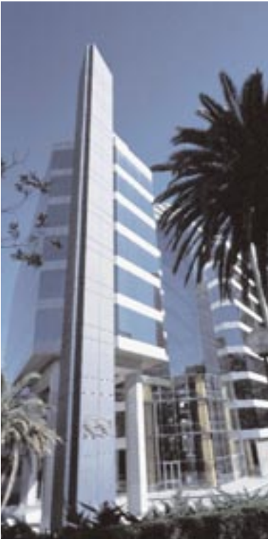
Building on calle Diagonal. Barcelona
