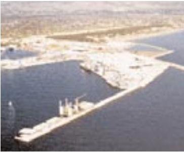
Remodelling the port of Castellón
