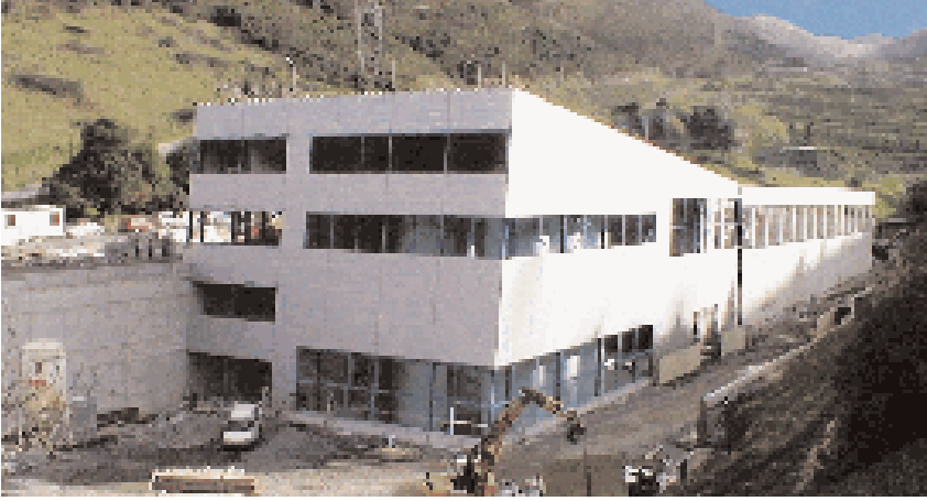
Leachate treatment plant in Artigas. Bilbao.
