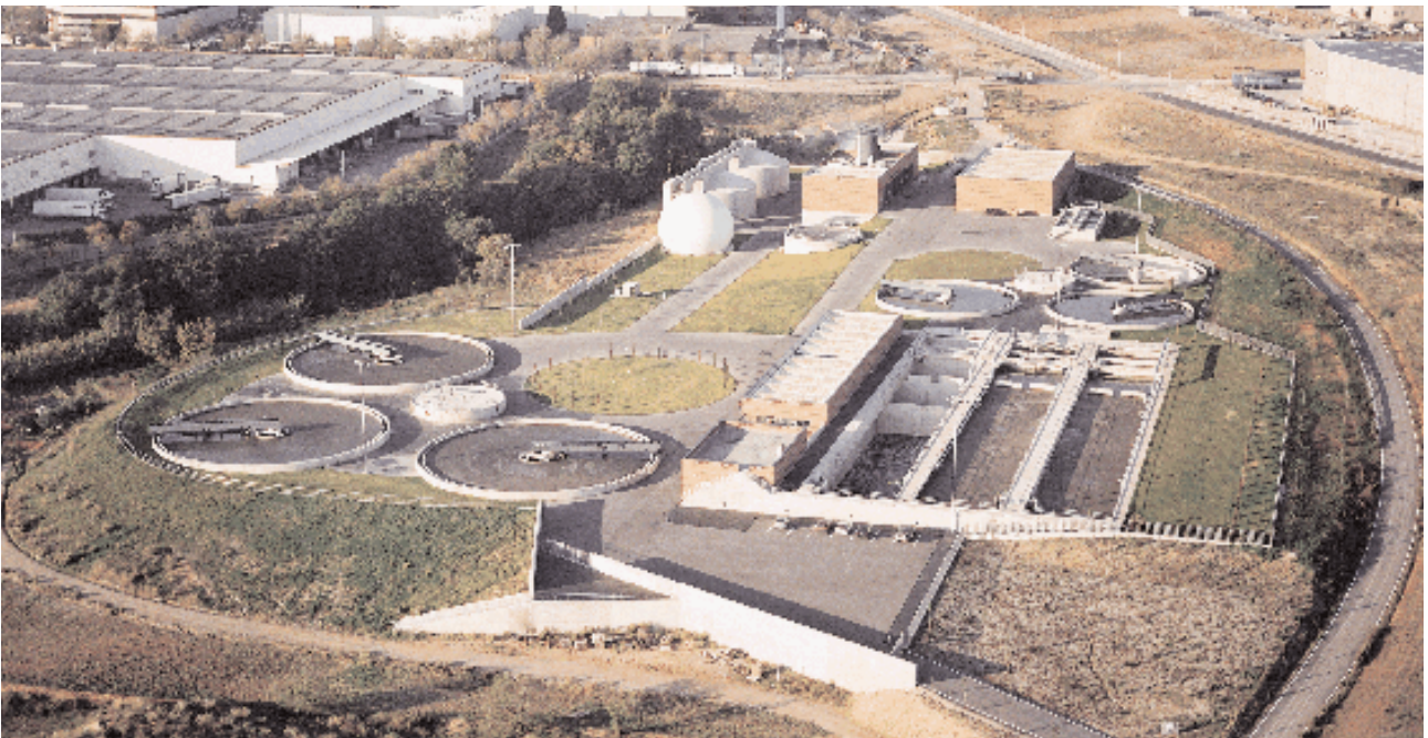
Wastewater purification station. Sabadell. Barcelona
