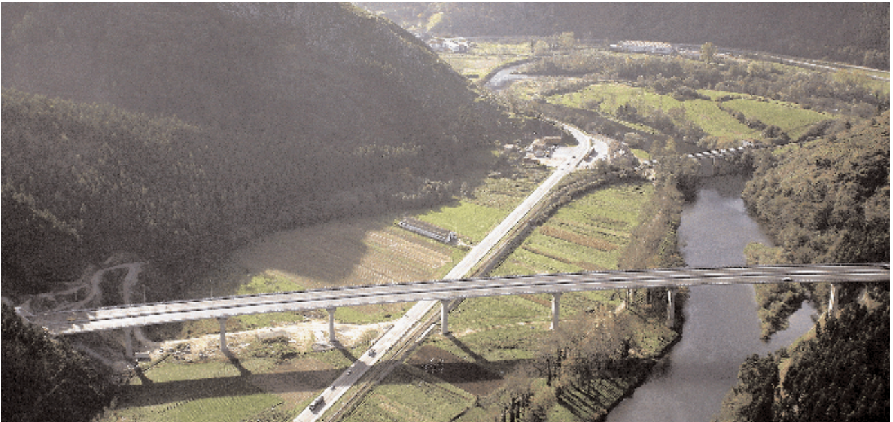
Autovía del Cantábrico, dual carriageway bordering the Bay of Biscay. Alternative route along the Sella River
