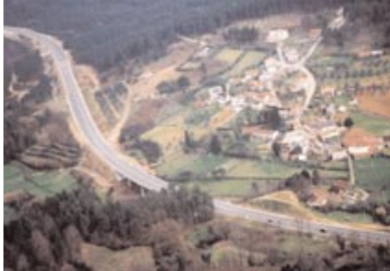
South Lisbon road. Viaduct over the Serrazela River. Portugal
