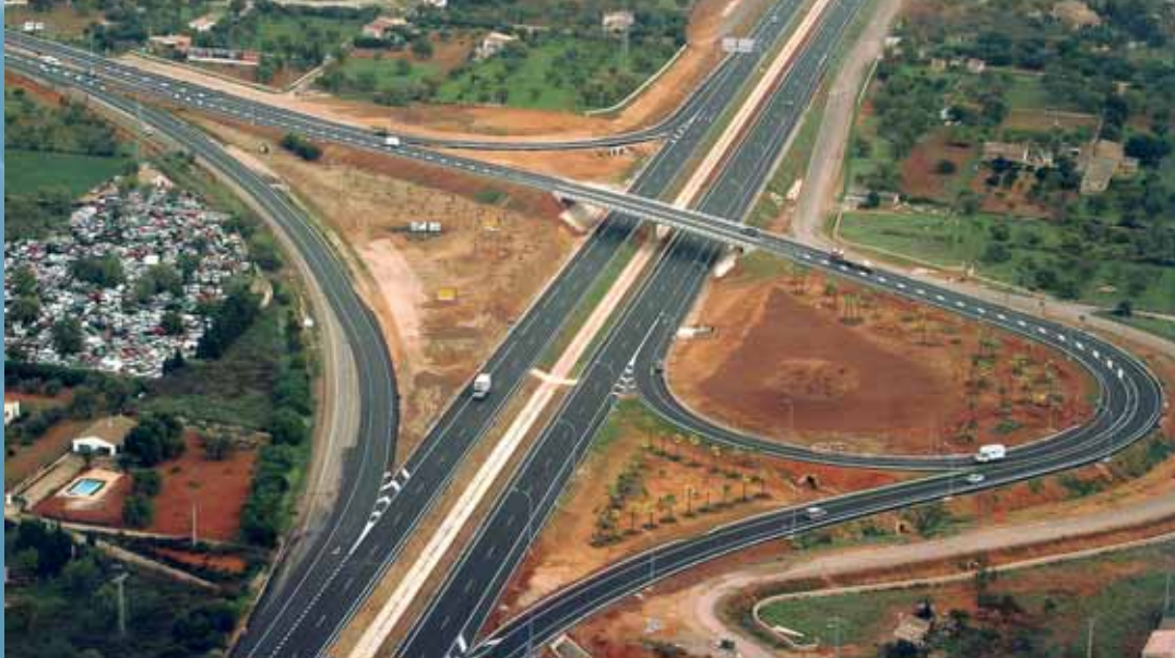
PM-27 central motorway, section III. Inca relief road. Mallorca
