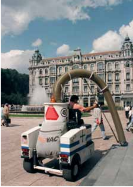
Sewer system maintenance. Oviedo
