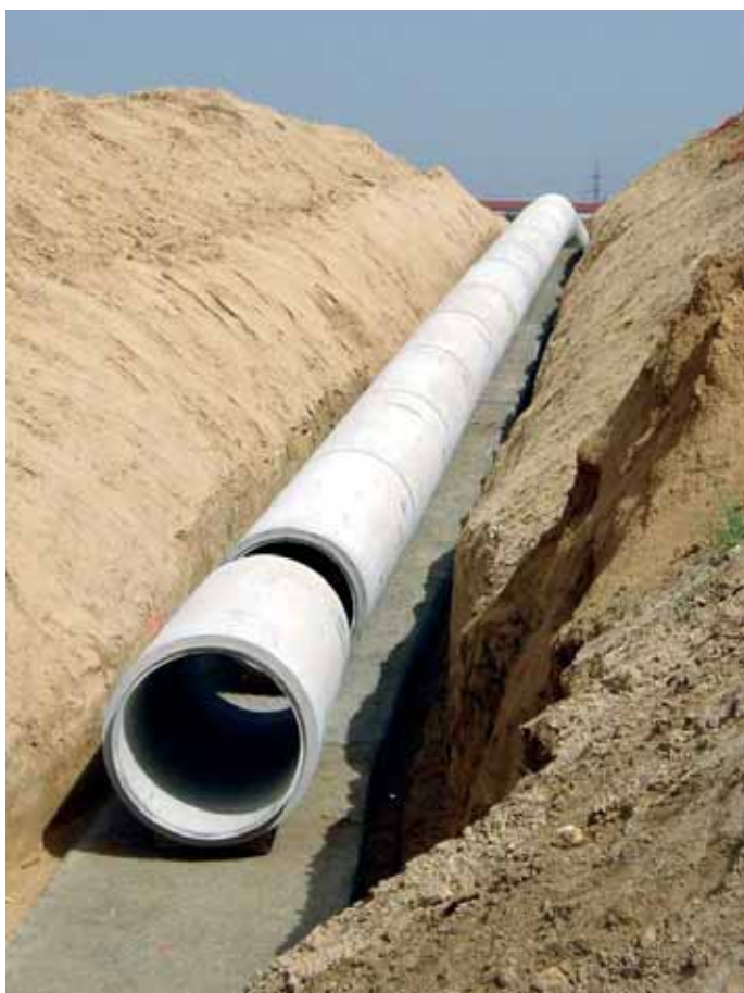
Poststressed concrete pipes with metal sleeves and elastic gaskets
