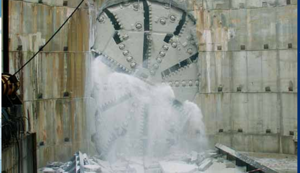
TBM on Line 9 of the Barcelona underground
