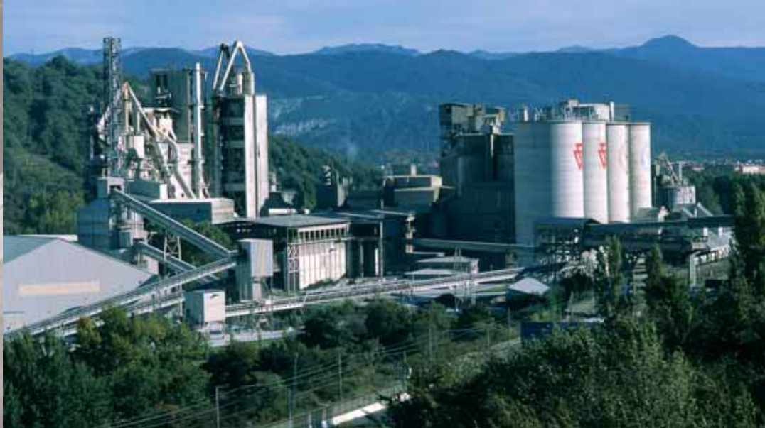
Olazagutía cement factory. Navarra
