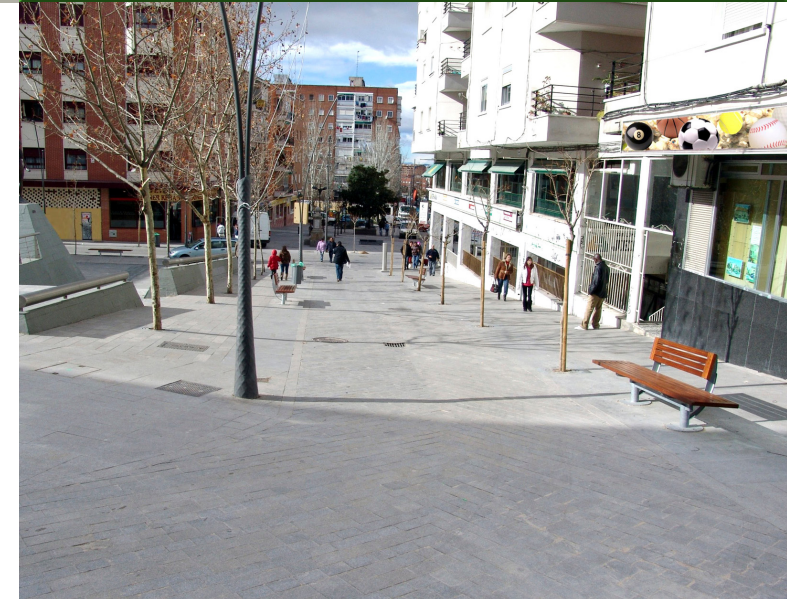
Remodeling of the central Alcorcón, Madrid.
