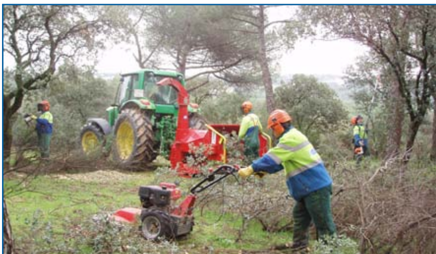
Crushing and clearing works
