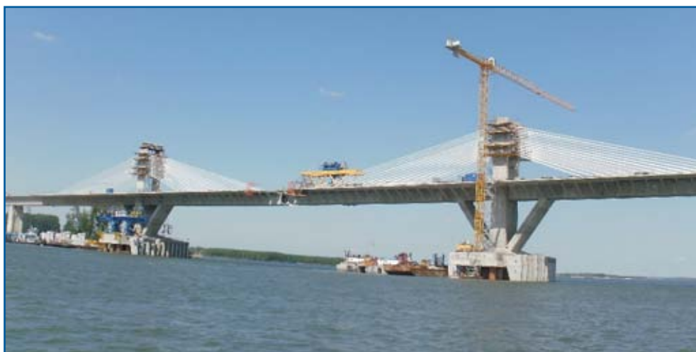
Vidin-Calafat Bridge (Bulgaria-Romania)
