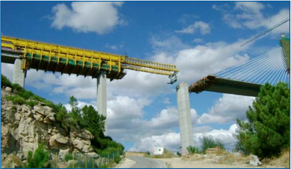
Corgo Viaduct, Portugal
