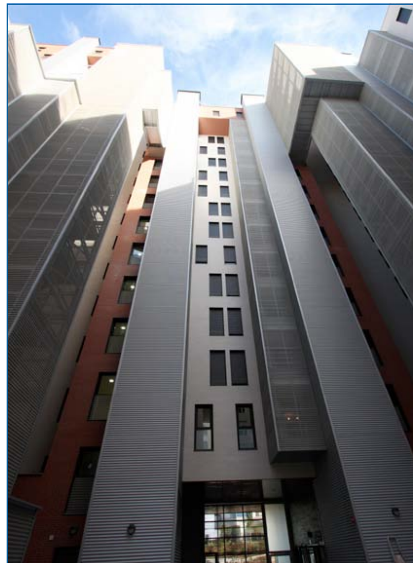
Homes in Móstoles (Madrid)
